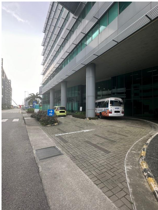
TOLL Bldg Main Entrance – Side View
