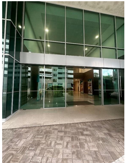
TOLL Bldg Main Entrance – Front View
